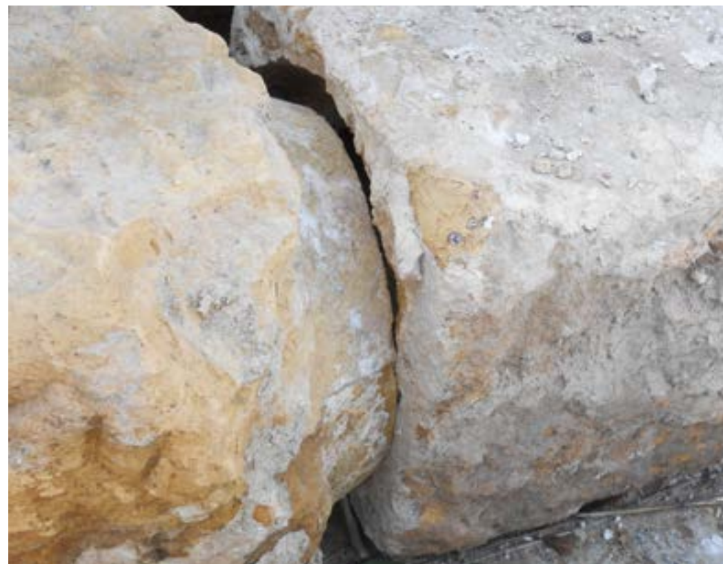
Between each part of the pipe there is a very thin layer of hydraulic limestone
